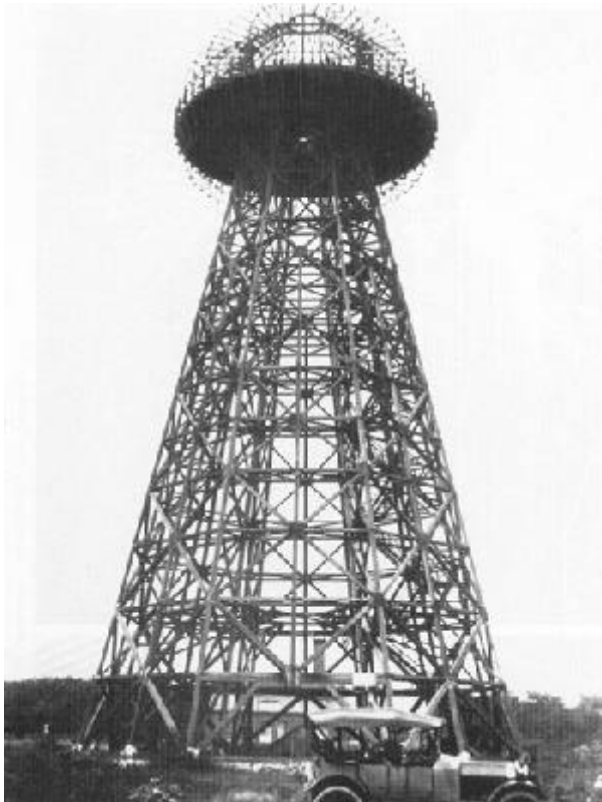
Figure 11: The skeleton of the first TESLA plant (constructed ~1901-1903) for the transmission of energy and broadcasting signals in Wardenclyffe, Long Islands, New York. It was never completed.
